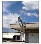
SM with passive reflector for long range connectivity
